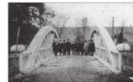
Figure 2: Contractor O. L. Hicks is second from left in this 1909 photograph (University of Toronto Archives, C. R. Young, B78-0001/007(14))
