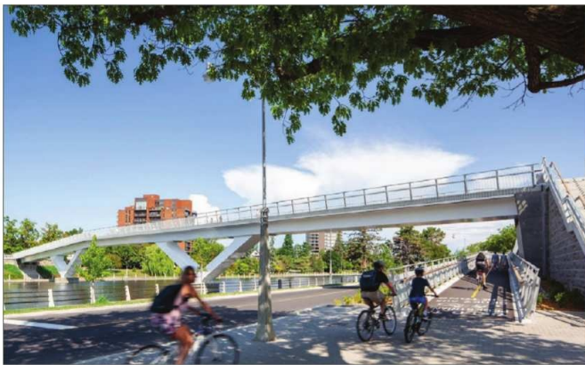
Figure 3: Flora Footbridge over Rideau Canal; a fully accessible structure 4 .
