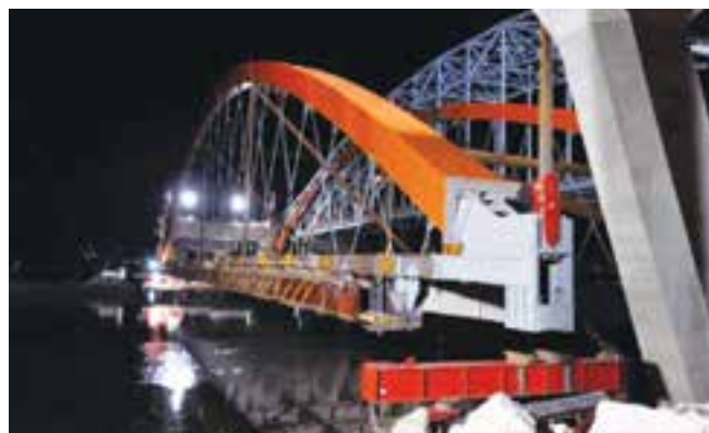
Figure 8. Hasting Bridge in Minnesota (PHOTO CREDIT: PARSONS CORPORATION)
