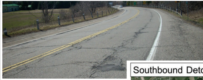
Left inset: Surface of Spragues Road in poor condition, May 2015. Facing page left: Spragues Road following unbonded concrete overlay, October 2015. Below: southbound traffic detour around project extents. Route shown in red denotes original route and length, while yellow denotes the route and length of the detour.
