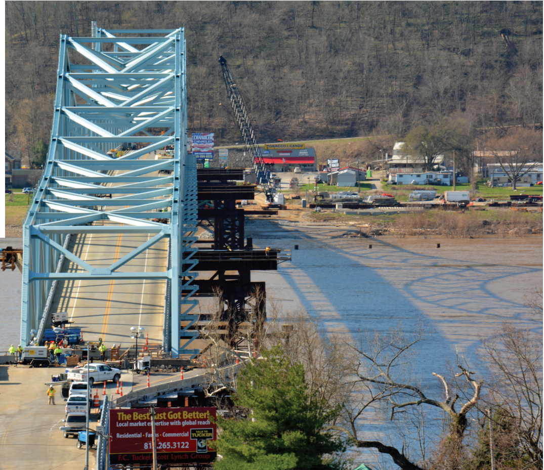
Above: Halfway there! The new bridge truss superstructure being slid laterally onto the rehabilitated piers of the original bridge beside it. Inset: New bridge superstructure being constructed on temporary supports while existing bridge carries traffic.
