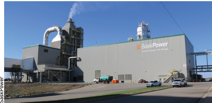
Exterior of CCS facility.
