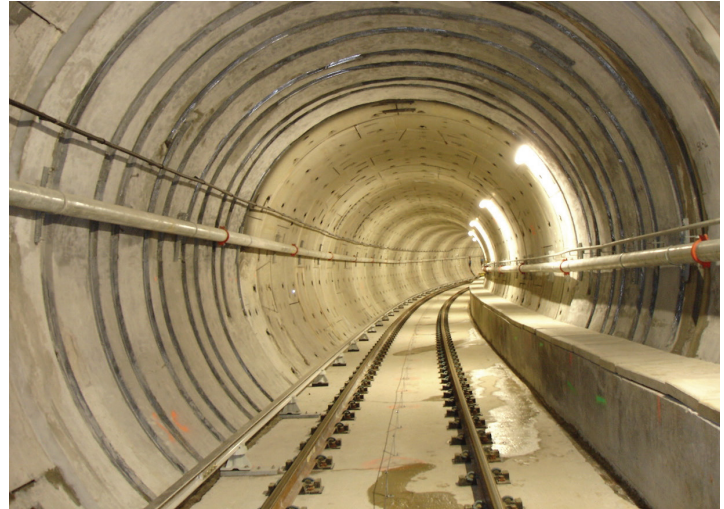
The construction of the Yaletown station on Canada Line. Right: A completed bored tunnel for the Canada Line rapid transit project.
