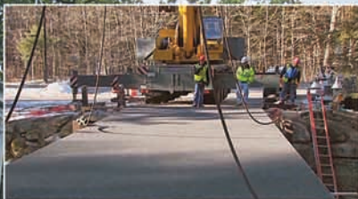
Deck installed in 30 minutes
