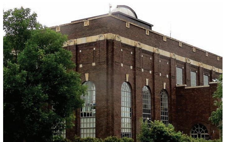
Powerhouse building in Regina as it looks today.
