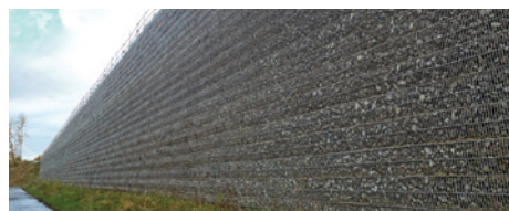
(Above) Approaching the new Port Mann Bridge. (Below) Owing to unstable slopes, poor soils and constrained rights of way, several kilometres of retaining walls were built, up to 10 metres in height.
