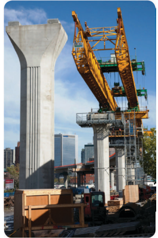
Elevated guideway construction.
