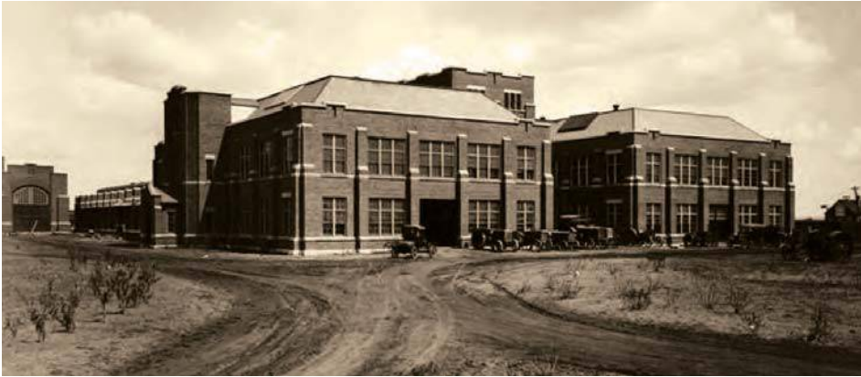
Figure 2: Engineering Building, University of Saskatchewan, 1921.
