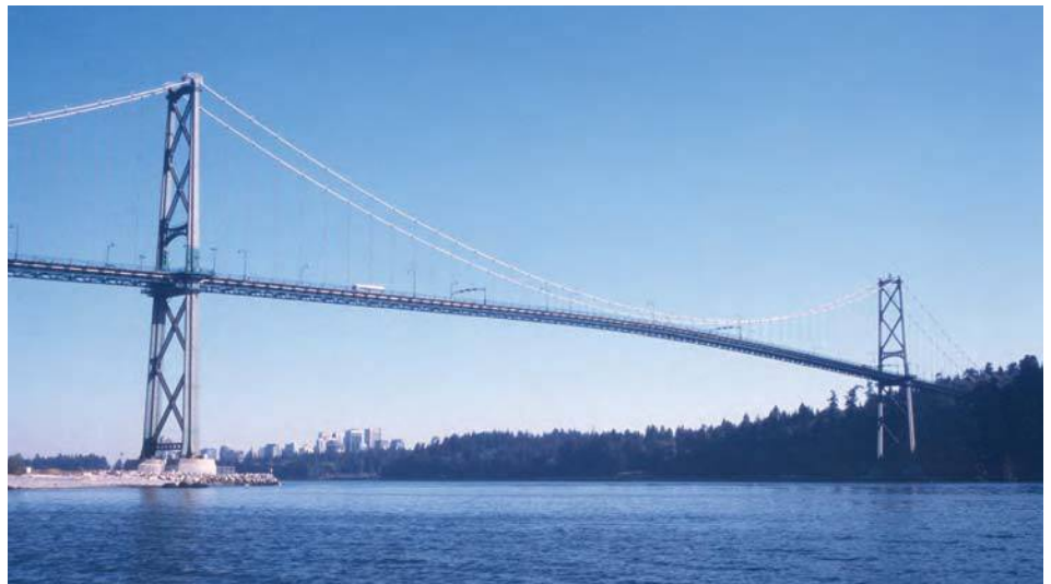
Lions' Gate Bridge, Vancouver: renovation
