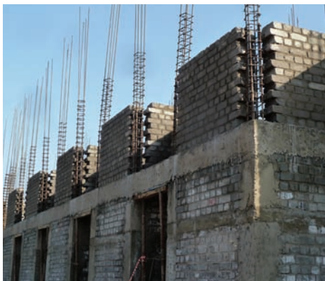
Figure 2. Confined masonry walls under construction at the IITGN Palaj campus.
