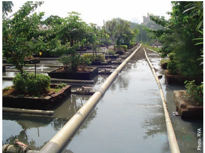
Above: operator's garden at Worli-Lovegrove being watered using the plant's effluent water.
