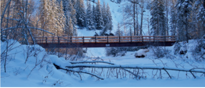
One of two bridges to the bonebed which lies in a steep valley. Construction had to be done quickly and during winter.
