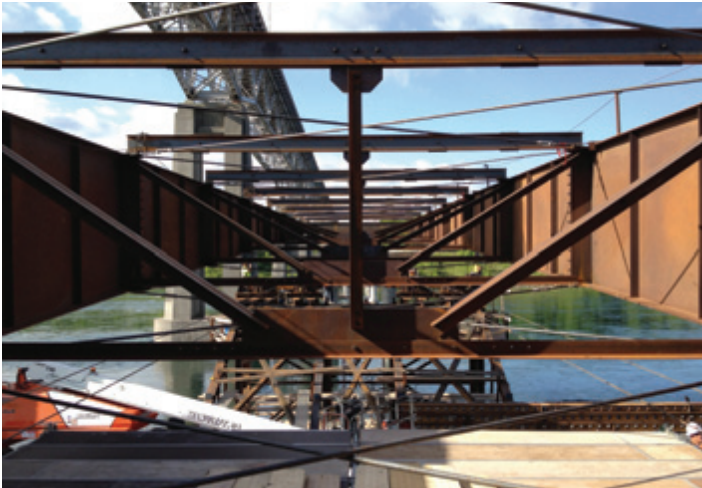
View from inside the launching nose in cantilever.
