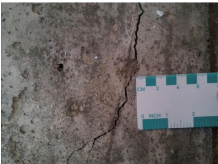
Figure 1: Vertical and map cracking observed in foundation walls of the affected houses. The map cracks are sealed to avoid water penetration and further damage.
