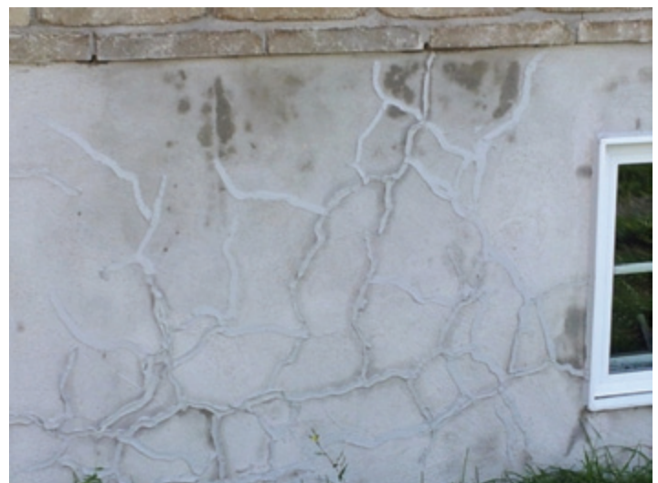
Figure 1: Vertical and map cracking observed in foundation walls of the affected houses. The map cracks are sealed to avoid water penetration and further damage.
