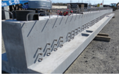
T-beam prior to installation.
