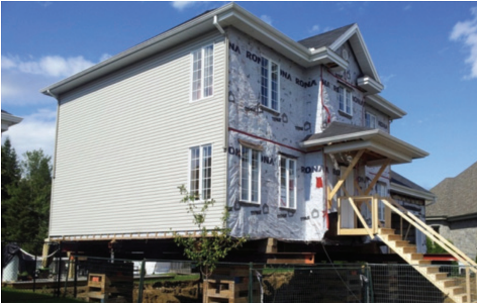
Figure 2: Replacement of foundation walls in severely deteriorated houses.
