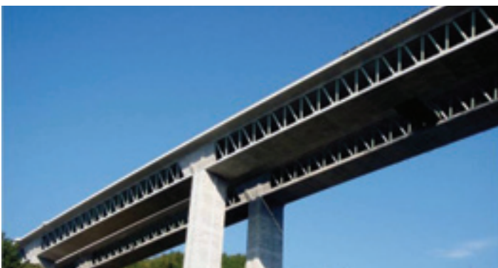
Photo 1 – Saruta River Bridge
