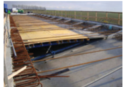
Figure 6 – Formwork of the overhangs
