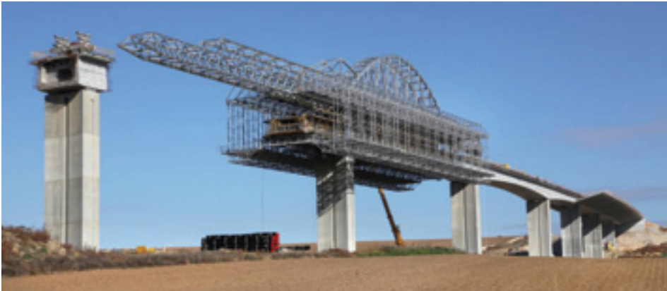
Figure 4 – Progressive erection of the bridge
