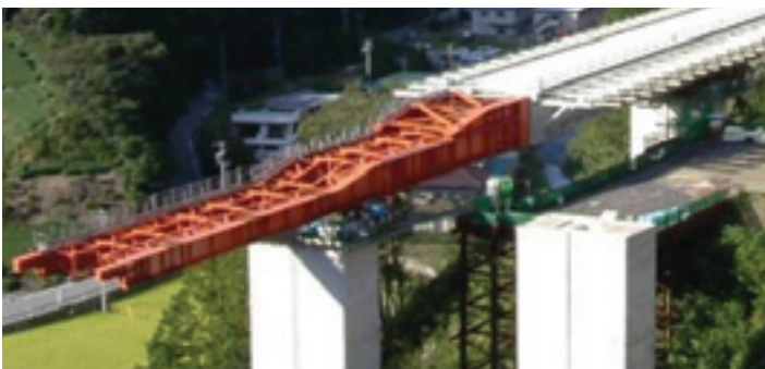
Photo 6 – Incremental launching erection of Katsurajima Viaduct
