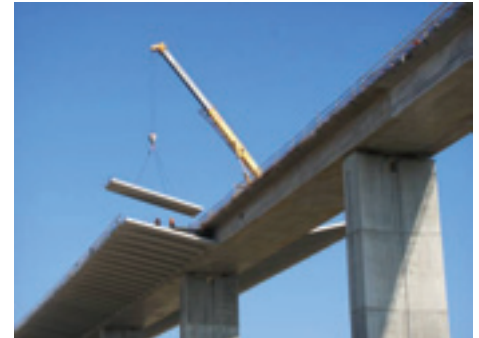
Figure 5 – Erection of precast struts
