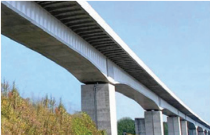
Photo 2 – New Akabuchi River Bridge
