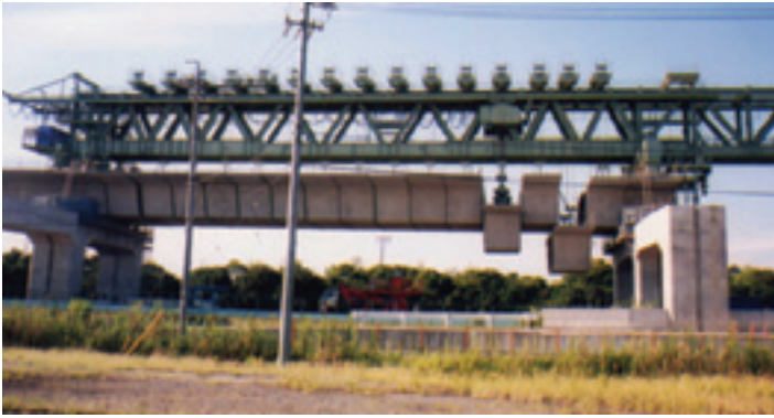
Photo 4 – Erection of the Yatomi Viaduct
