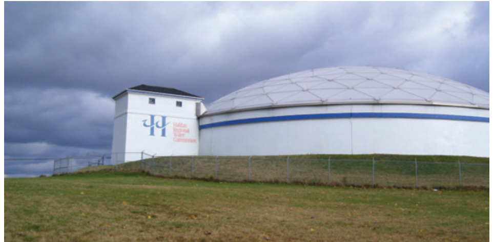
The Robie Street Reservoir in the north end of Halifax today, with its new geodesic lightweight roof installed in 2000. Halifax Water
