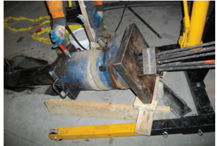
Tensioning jack on top of gate applying 250,000 lbs. of tension to the new grouted DCP post-tensioned trunnion anchors which are located about 8 ft. below.
