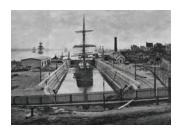
The graving dock was opened in 1889. It was then the largest dry dock on the eastern seaboard and could accommodate the largest vessels of the day. It is 173 m long x 24 m wide x 9 m high. The graving dock was built completely in the dry, using an earthen
