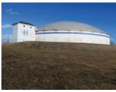
The 48 m diameter x 7.5 m deep concrete reservoir was originally built in 1913. It was one of the few structures in the area to survive the Halifax explosion in 1917, less than 1 km away. Deterioration to the walls and roof required extensive
