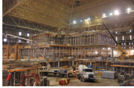
(Left) Demolition of the former hockey arena gets under way; the interior was gutted, including the seating bowl which had provided lateral stability to the exterior walls. (Centre) Construction of a concrete frame within the interior. (Right) Shoppers browse in the new grocery store.
