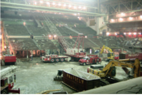
(Left) Demolition of the former hockey arena gets under way; the interior was gutted, including the seating bowl which had provided lateral stability to the exterior walls. (Centre) Construction of a concrete frame within the interior. (Right) Shoppers browse in the new grocery store.
