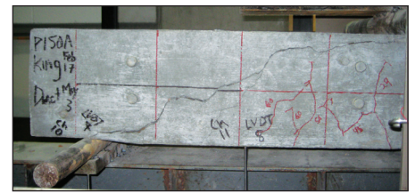
FIGURE 5: Typical shear failure of precast slab-beam specimens
