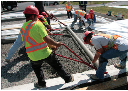
FIGURE 2: Hydraulic roller screed running along pervious concrete and curb & gutter.
