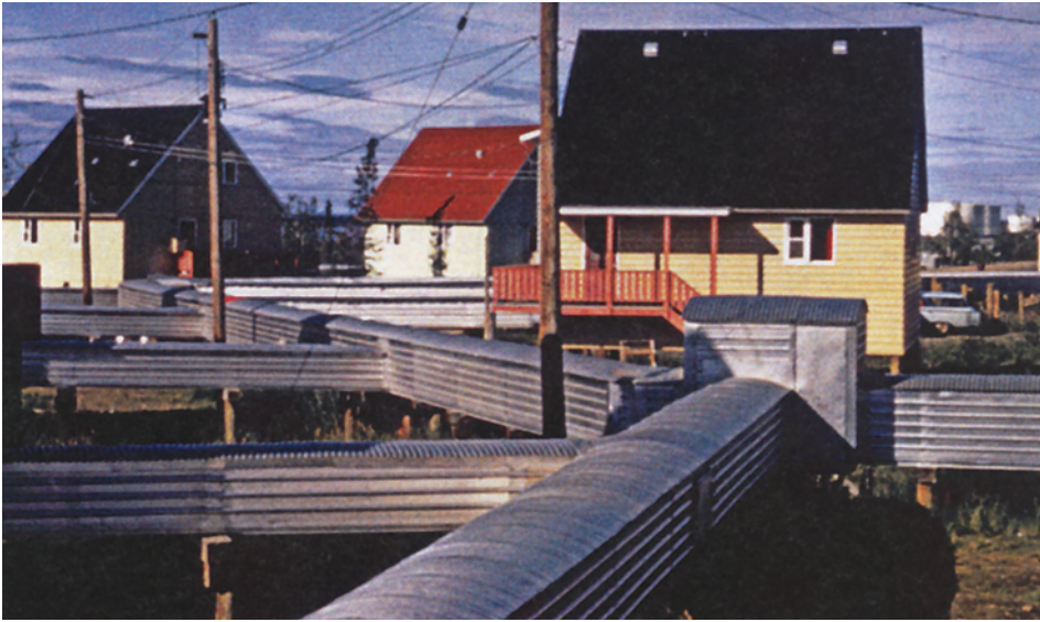
Inuvik's above-ground "utilidor" prevents water and sewer pipes from warming the permafrost.
