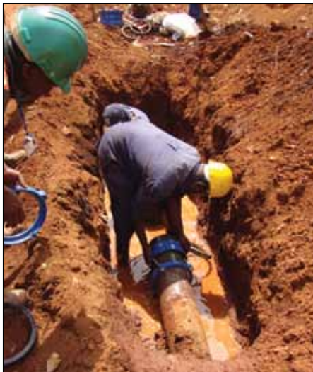
FIGURE 2: Repairing watermain.
