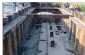
Steel Piles Driven
