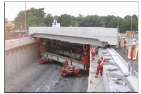
FIGURE 7: New Island Park WB Superstructure.
