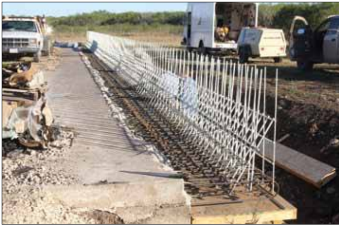
FIGURE 12: Views of the Arrangement of GFRP Reinforcement in the Tested Barrier Before Concrete Casting.
