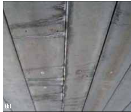
FIGURE 6: Types of Distress in Adjacent Box-girder Bridges. (a) Water Leakage through the Joint (b) Efflorescence on Joint Underside (c) Concrete Spalling and Steel Rusting
