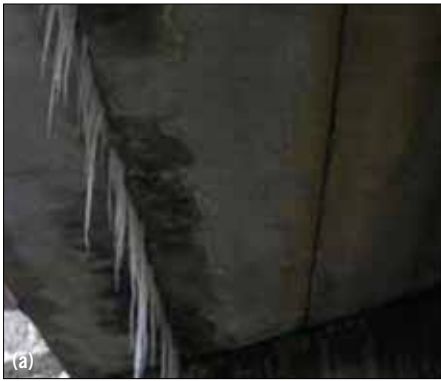
FIGURE 6: Types of Distress in Adjacent Box-girder Bridges. (a) Water Leakage through the Joint (b) Efflorescence on Joint Underside (c) Concrete Spalling and Steel Rusting
