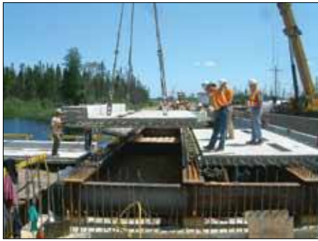
FIGURE 5: Installation of Full-Depth Deck Panels.
