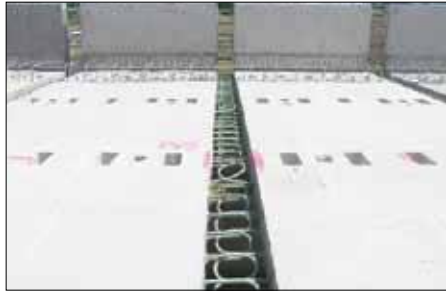
FIGURE 10: Closure Strip & Shear Pockets.
