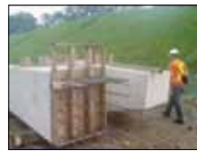
Precast Pier Cap
