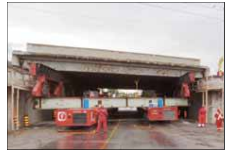
FIGURE 8: SPMT's at Existing Clyde Avenue Bridge.
