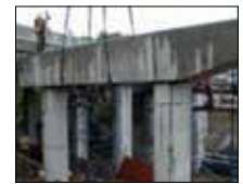
Pier Cap Installed
