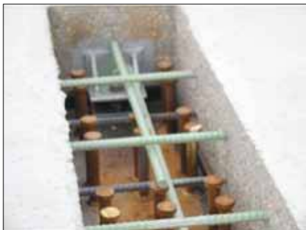
FIGURE 7: Shear Studs in Preformed Pockets.
