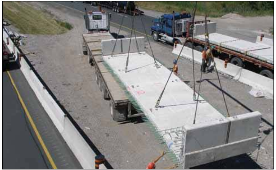
FIGURE 8: Precast Panels Lifted from Truck.
