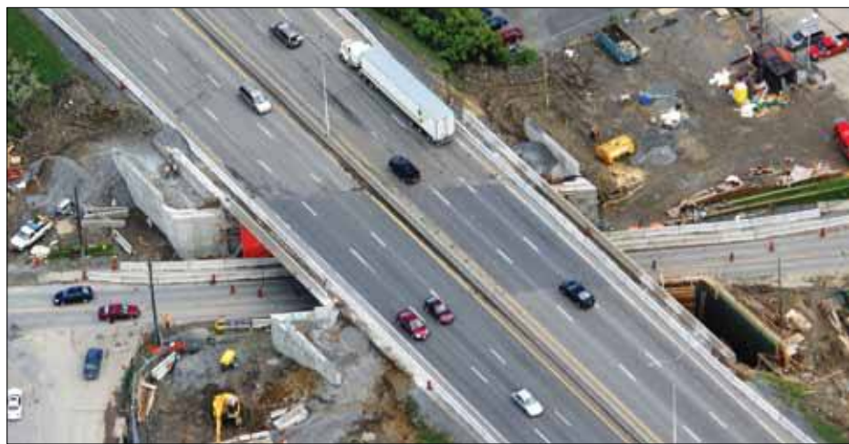
FIGURE 2: Clyde Avenue Overpass.
