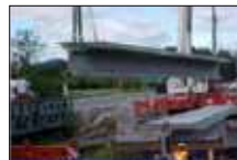
Precast Beam Installed
