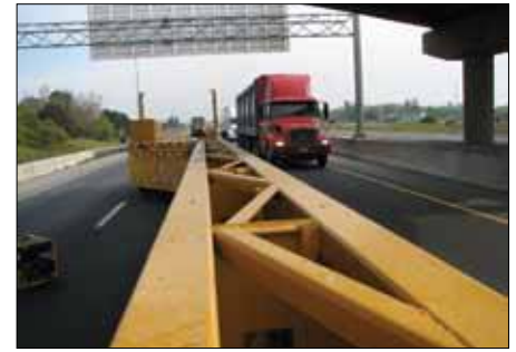
FIGURE 10: Mobile Barriers Trailer in use at the Dingman Drive Bridge.
