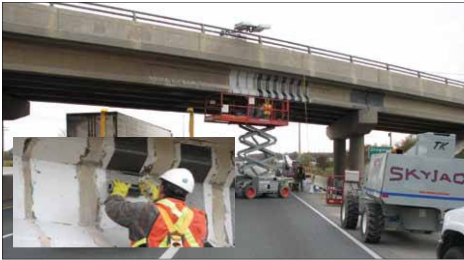
FIGURE 9: Application of CFRP Strips with a Roller.
