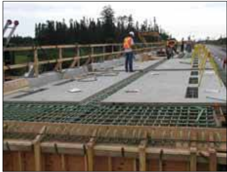
FIGURE 6: Closure Strips between Deck Panels.
