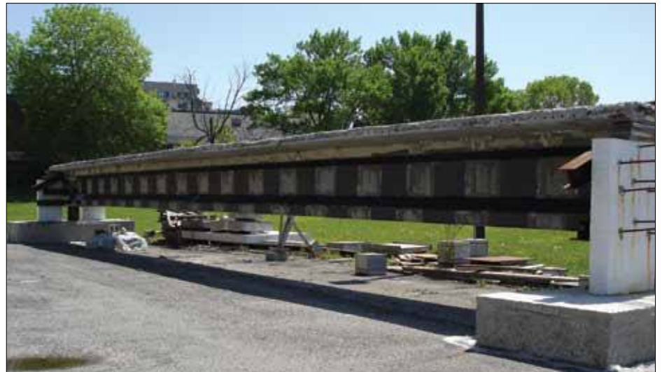
FIGURE 3: Final View of the Girder after Application of CFRP Sheets.
