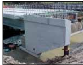
FIGURE 3: Precast Wingwall Unit.
