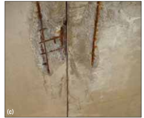
FIGURE 6: Types of Distress in Adjacent Box-girder Bridges. (a) Water Leakage through the Joint (b) Efflorescence on Joint Underside (c) Concrete Spalling and Steel Rusting
