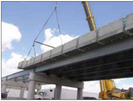
FIGURE 9: Installation of Full-Width Deck Panels.
