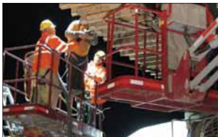
FIGURE 8: Workers Pumping Self-consolidating Concrete to Reinstatement Damaged Girder.
