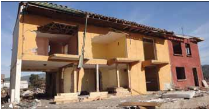
FIGURE 1: Residential Structure in Pellhue, Chile.
