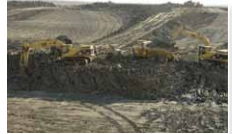
Above: Over the course of the floodway project, approximately 21 million cubic metres of earth were excavated from the floodway channel, which more than doubled the capacity of the floodway from 60,000 to 140,000 cfs. / Pendant l'exécution des travaux, environ 21 millions de mètres cubes de terre seront déplacés du lit du canal afin d'en doubler la capacité, qui passera de 60 000 à 140 000 pi 3 /s cfs.
