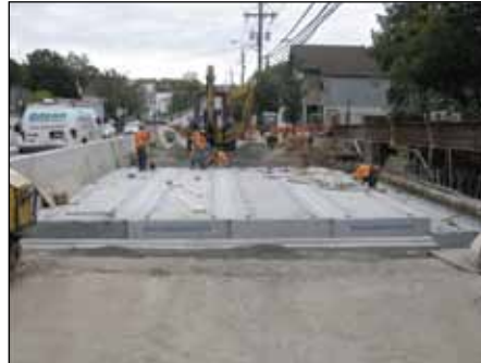
FIGURE 5: HCB Planks Ready for Deck.
