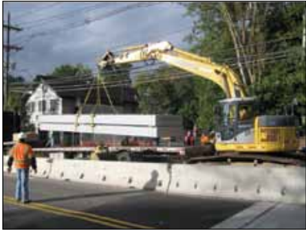
FIGURE 4: Picking 2 HCB's with Excavator.
