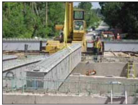
FIGURE 3: Erecting HCB with 30 tonne Crane.
