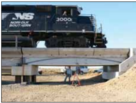
FIGURE 2: Live Load Test—Railroad Bridge.
