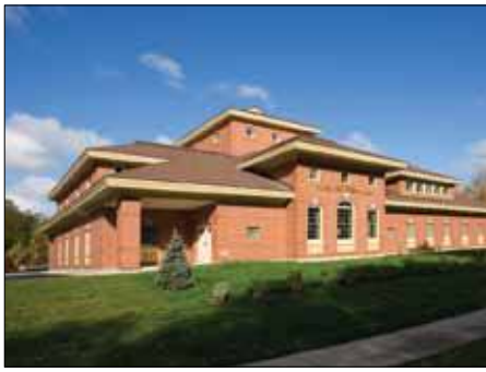
ABOVE: Bliss Water Treatment Plant.
