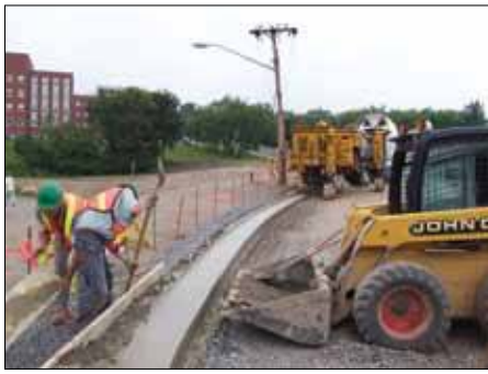
ABOVE AND RIGHT: Installing new infrastructure in Fredericton.
