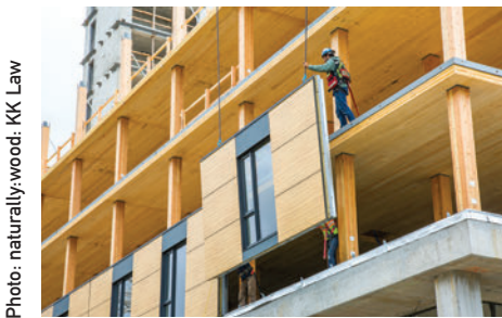
UBC's Brock Commons under construction
