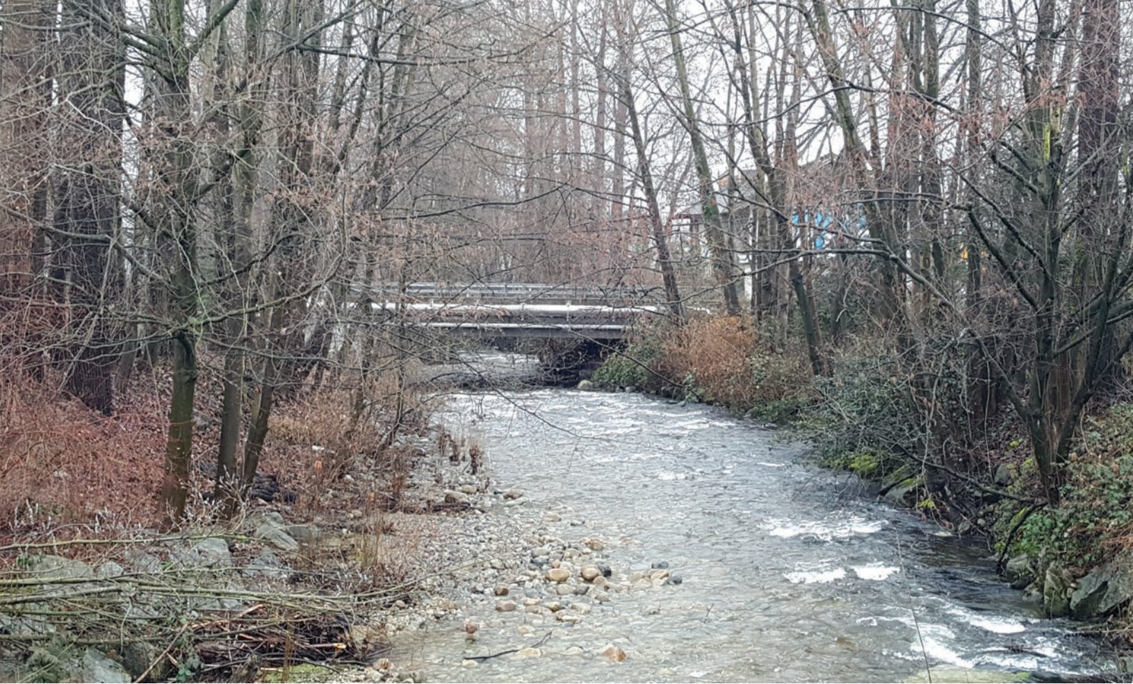
Mosquito Creek Bridge, North Vancouver
