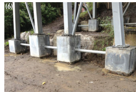
(1) Mission Bridge, B.C., seismic retrofit under construction, and (4) pier jackets completed. (2) CN Rail bridge, Montreal, pier jacking during construction, and (3) repairs completed. (5) Hagwilget Bridge, Hazelton, B.C., forming details and reinforcement for steel bent leg encasements, and (6) UHPC encasements before capping.
