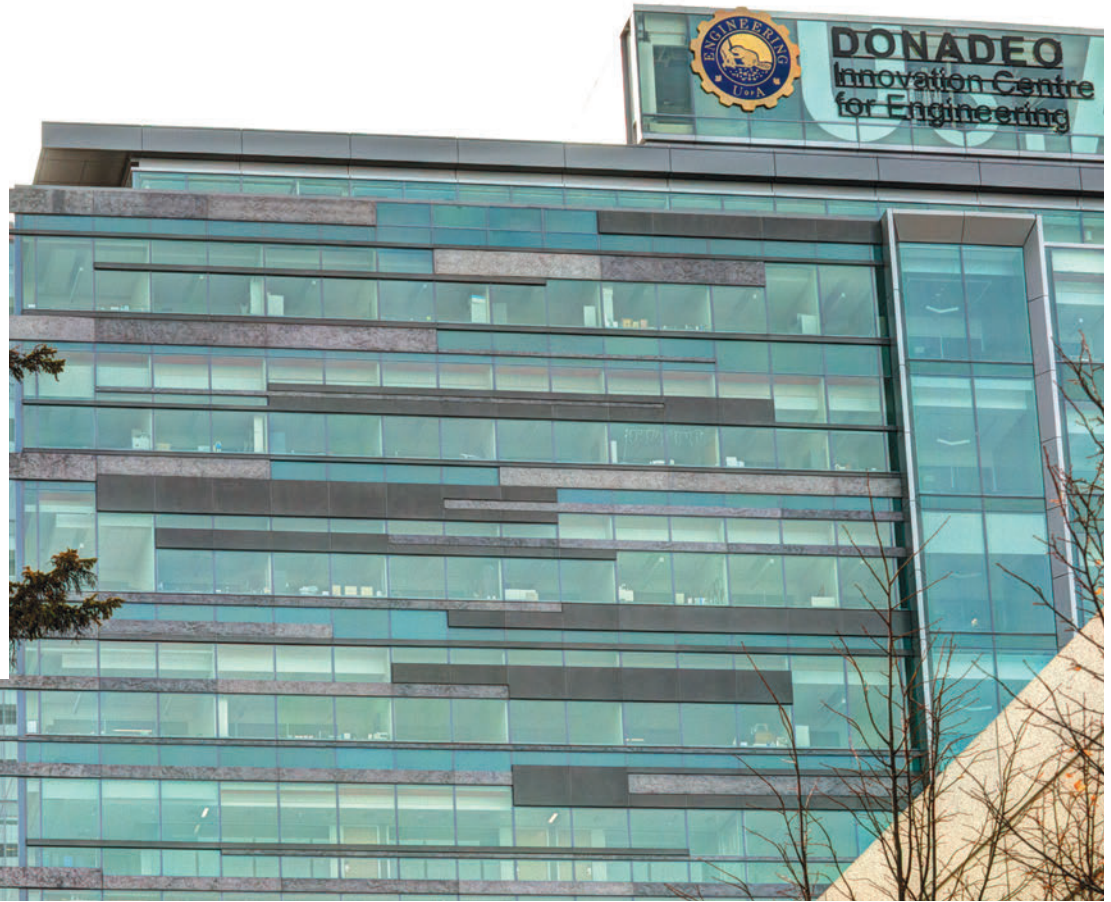
Top left: Fly-by corners. Above: The building façade combines glass, metal, and UHPC panels. Far left: Panel texture resembles stone in appearance. Left: Assortment of UHPC panels after casting.
