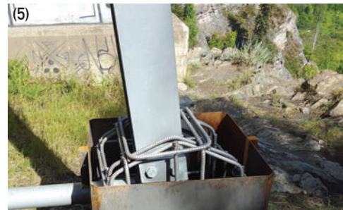
(1) Mission Bridge, B.C., seismic retrofit under construction, and (4) pier jackets completed. (2) CN Rail bridge, Montreal, pier jacking during construction, and (3) repairs completed. (5) Hagwilget Bridge, Hazelton, B.C., forming details and reinforcement for steel bent leg encasements, and (6) UHPC encasements before capping.
