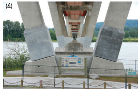
(1) Mission Bridge, B.C., seismic retrofit under construction, and (4) pier jackets completed. (2) CN Rail bridge, Montreal, pier jacking during construction, and (3) repairs completed. (5) Hagwilget Bridge, Hazelton, B.C., forming details and reinforcement for steel bent leg encasements, and (6) UHPC encasements before capping.
