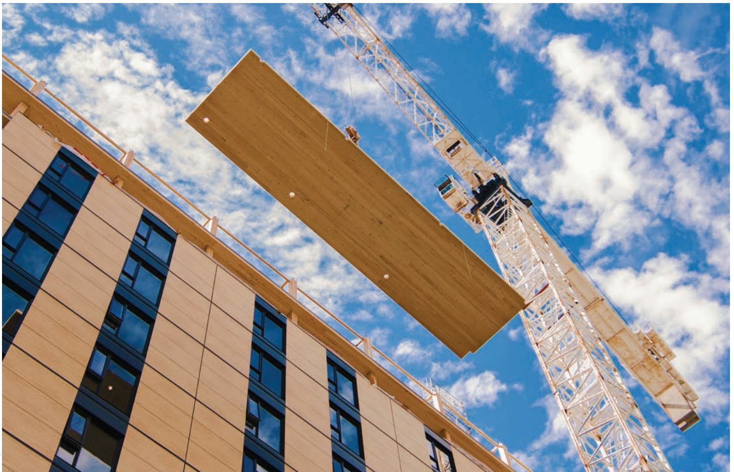
Figure 1: Timber erection – summer 2016. (Right) Figure 2: Point supported CLT system
