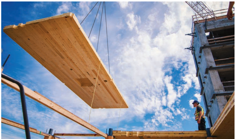
Top, Figure 5: Braced columns Middle, Figure 6: CLT panel installation Bottom, Figure 7: Perimeter envelope installation
