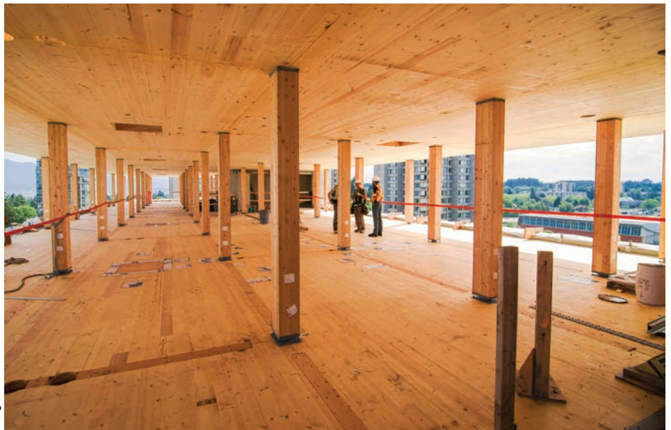
Figure 1: Timber erection – summer 2016. (Right) Figure 2: Point supported CLT system
