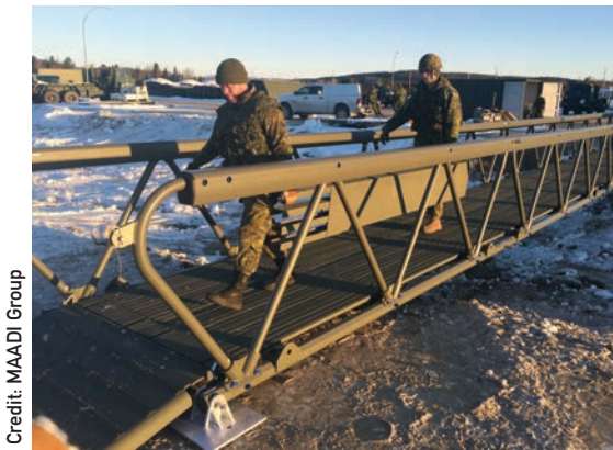
A rapidly deployable military bridge for the Canadian armed forces
