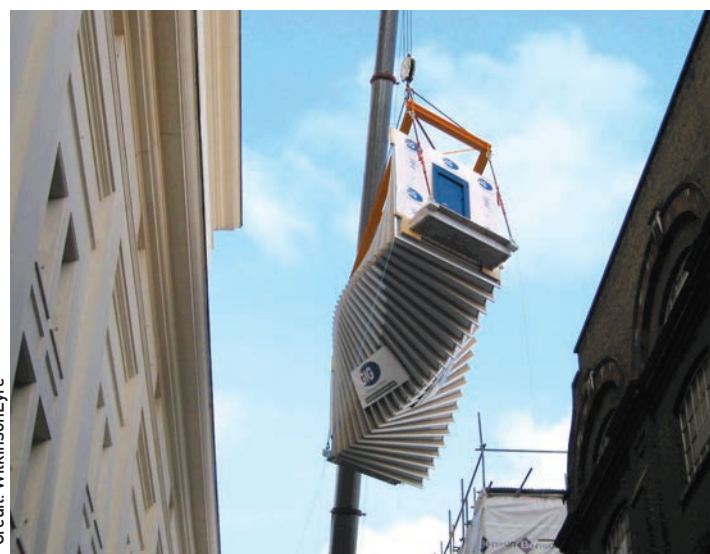
Bridge of Aspiration, London, UK, installation.
