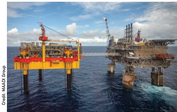
Pedestrian bridge linking an oil-rig and its accommodation platform.
