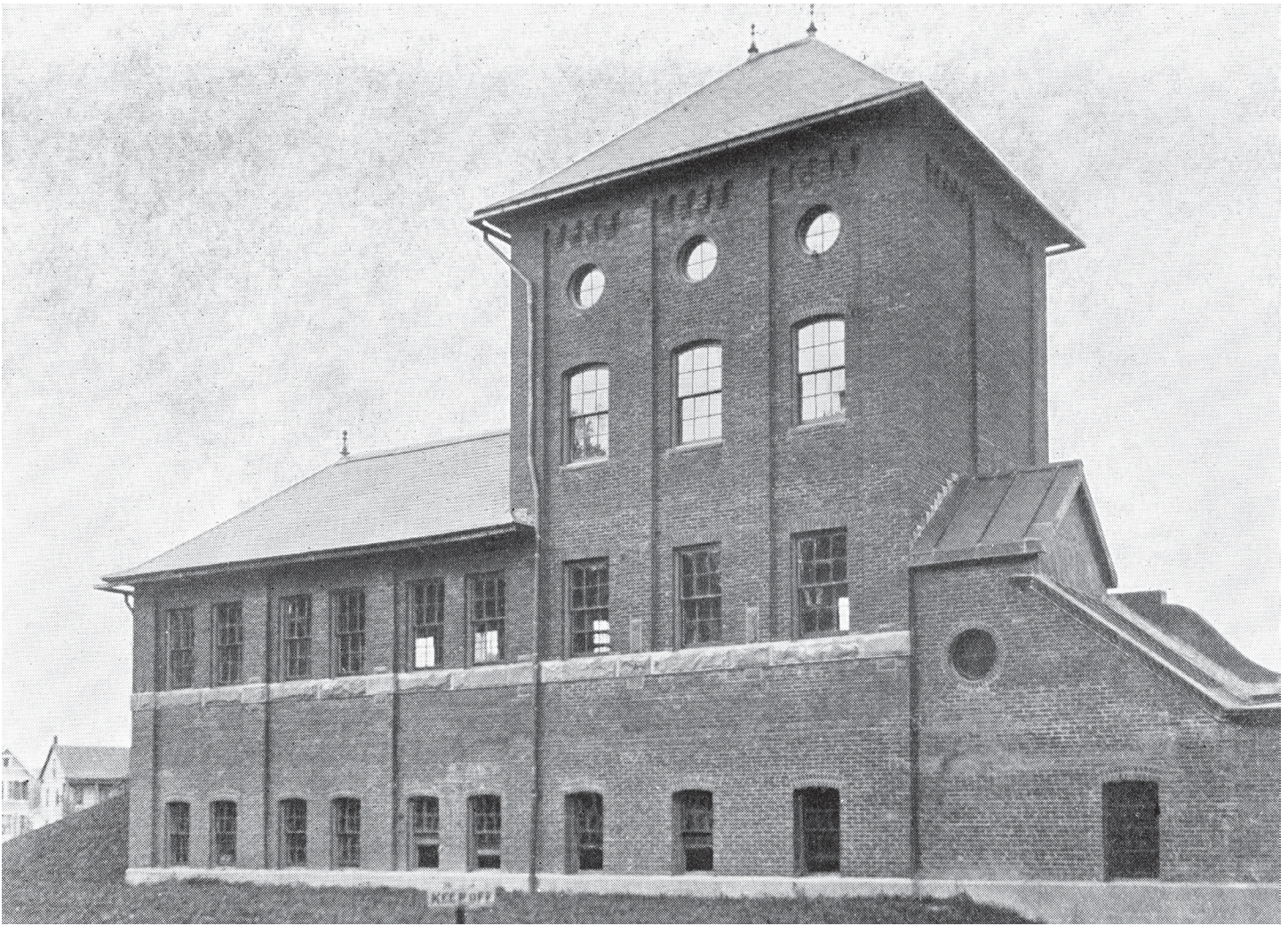
Fredericton Pumping Station and Water Treatment Facility (c 1906). The tall tower houses the constant head tank for backwashing the rapid sand filters located in the lower portion of the building. [Source: Provincial Archives of New Brunswick Image: P657-26]
