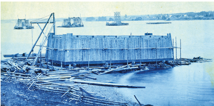
Figure 4: Timber caisson constructed on land prior to being floated into place and sunk, circa 1872 (Provincial Archives of New Brunswick, P119 Frank Sayer collection, P119-MS2I-109).
