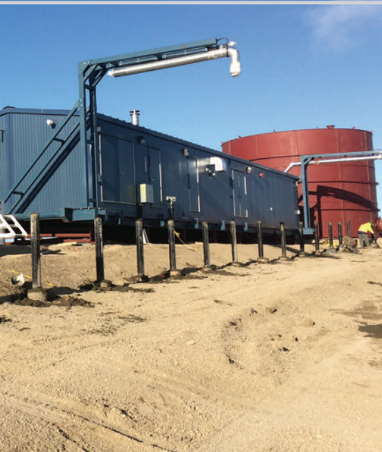
Far left: part of the packaged water treatment system being lifted onto piles. Left: backwash tank (yellow), water treatment plant, and potable water storage tank (not yet insulated).
