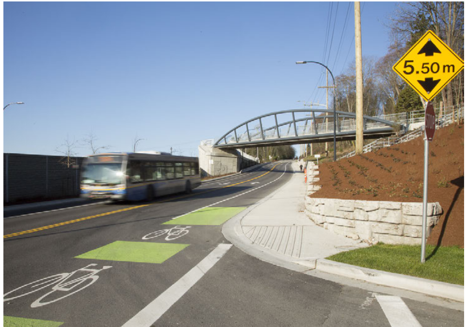
Pedestrian overpass at E 3rd Street
