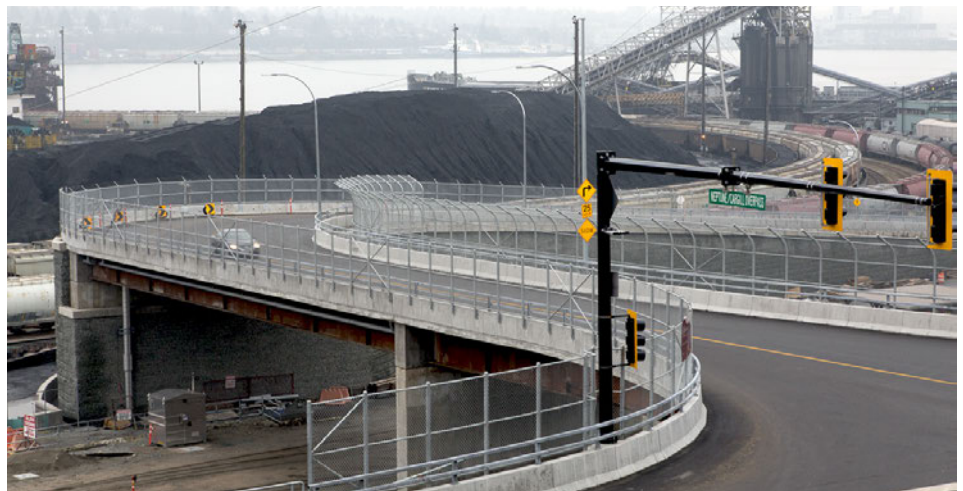
New overpass at Neptune/Cargill terminal entrance.
