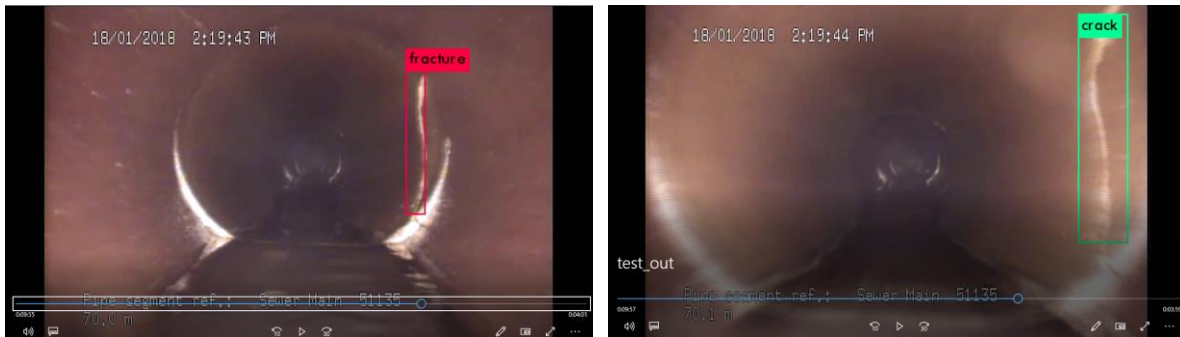
(b) Labeling of the same defect twice with two types of classification
