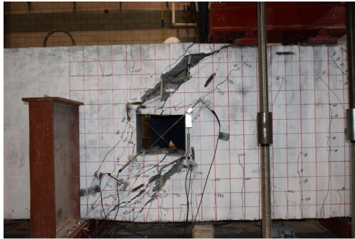
Figure 3: Typical Failure of deep beams with web openings (GO1)
