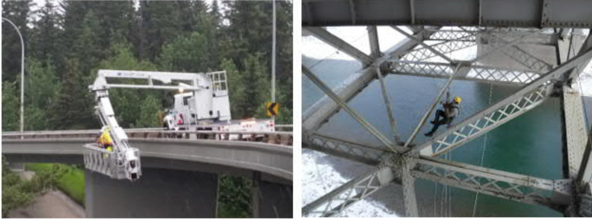
Figure 3: Recent Inspections completed using Snooper Truck and Rope Access
