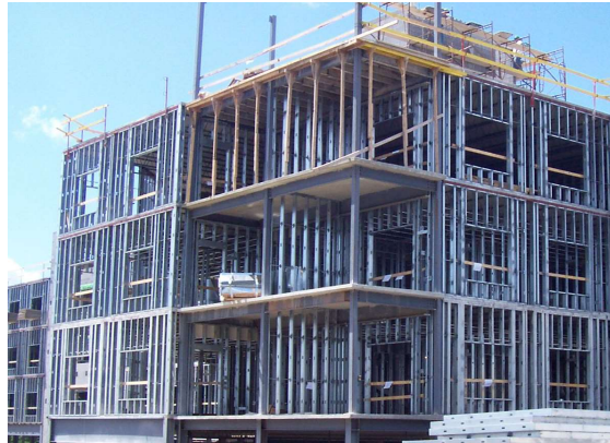
Figure 1 Cold-formed Steel Building
