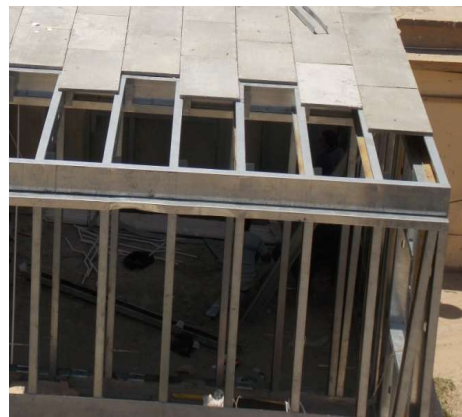
b) Erected Slabs
