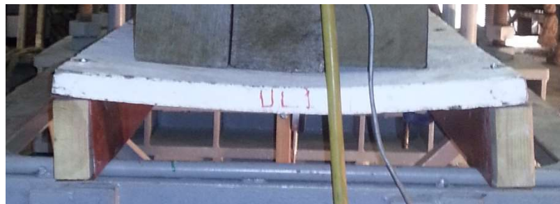
Figure 14 Slab Deflection and Mesh Failure at Ultimate Uniform Load
