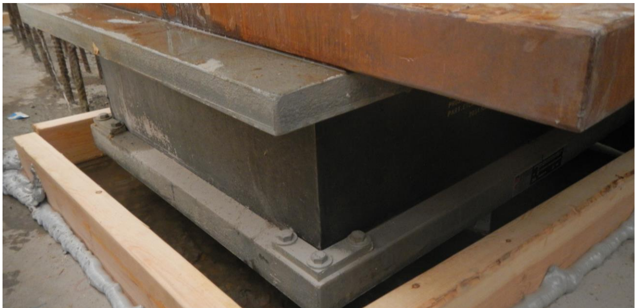
Figure 7: Elastomeric Bearing Pad in a Bridge Bearing
