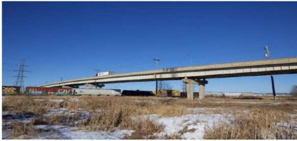
Figure 2: Large span bridge in Thunder Bay
