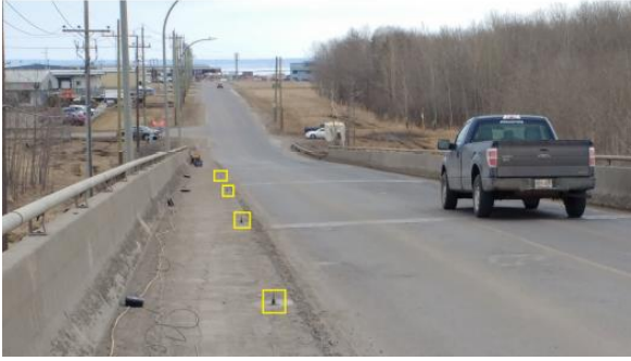
Figure 6: Sensors and DAQ placed on the sidewalk
