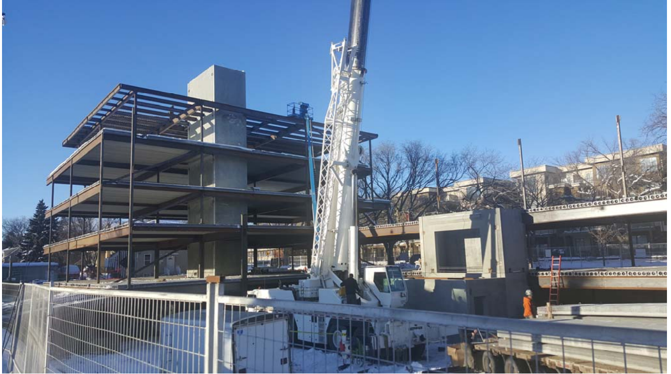
Figure 4 – Construction Site with Limited Unloading Area
