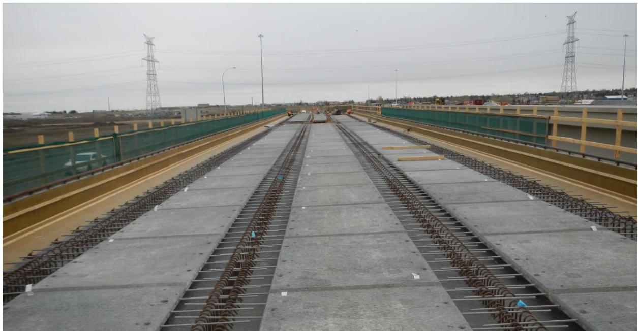
Figure 8: Precast and Prestressed Concrete Panels on Bridge Deck
