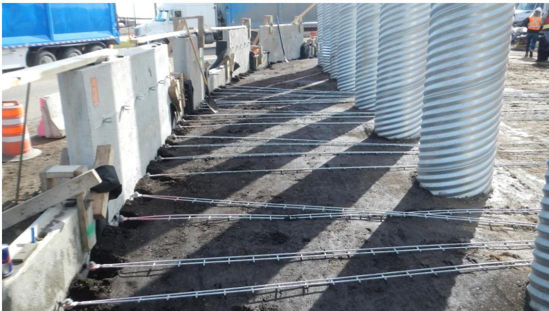
Figure 4: MSE Wall Back Fill Reinforcement
