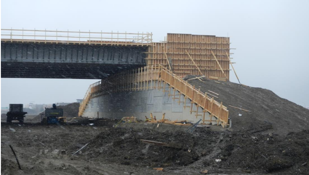
Figure 3: Mechanically Stabilized Earth (MSE) walls Designed as Bridge Abutments
