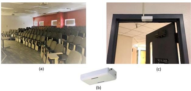
Figure 2: (a)Lecture hall under study, (b) EBTRON: CENCUS-C100 (c) Installed sensor on door frame
