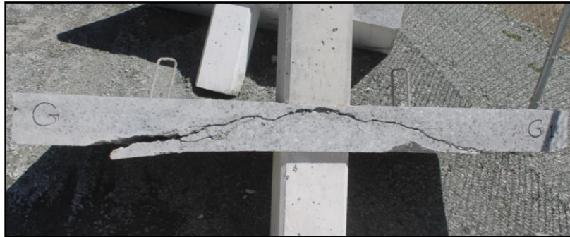
Figure 6: Saw-cut along the load direction.
