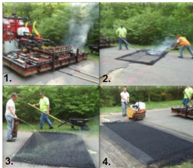
Figure 3: 1) Infrared Heating 2) Scarifying 3) Rejuvenators Added 4) Compaction (Kieswetter, 2013)
