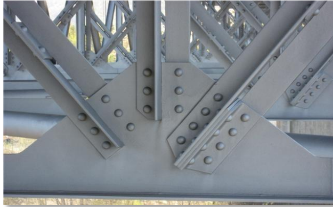
Figure 4 - The Rombak bridge in 2009 (Knudsen, 2012)
