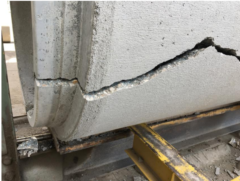
Figure 8: Cracking of specimen with single elliptical steel cage
