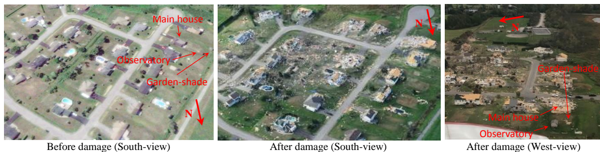
Figure 1: Aerial view of case-study neighbourhood before and after tornado damage
