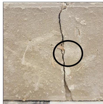
b) Fibre bridging flexural crack
