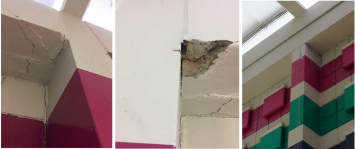
Figure 4: Natatorium precast beams and columns
