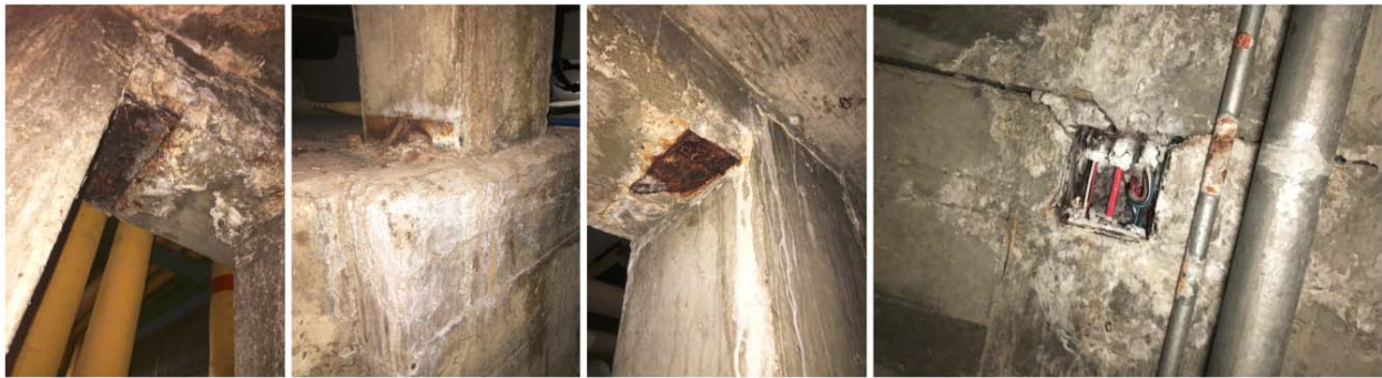
Figure 3: Tunnel deterioration
