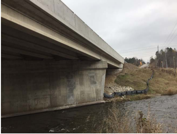
Figure 2: CPCI I-Girder semi-integral abutment bridge
