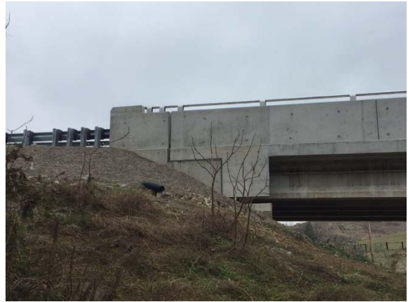
Figure 3: End diaphragm of completed bridge
