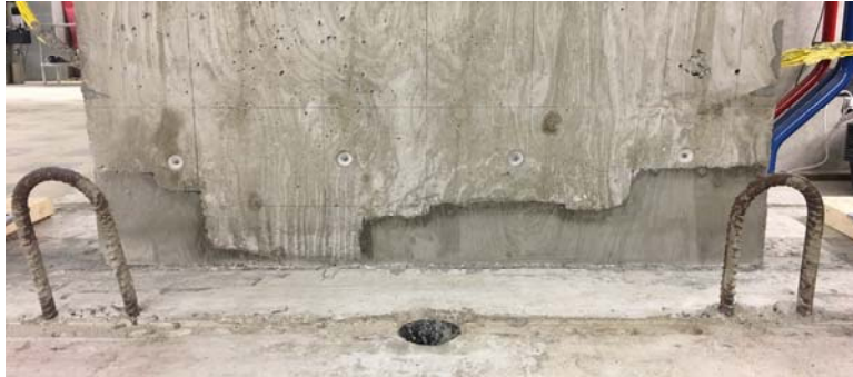
Figure 4. Repaired steel-reinforced wall.
