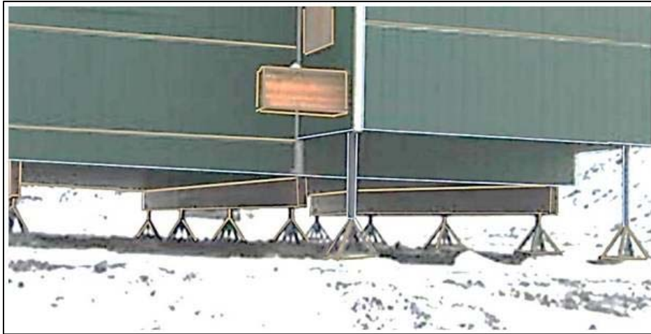
Figure 1: Typical Screw Jack Foundation System
