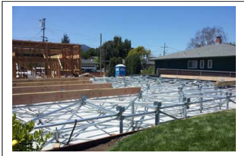
Figure 12: Tubular foundation frame and slab
