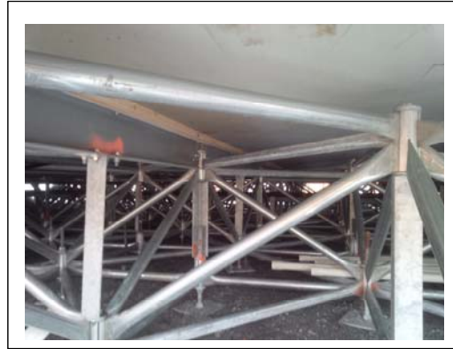
Figure 21: Assembled frame work showing beam support line.
