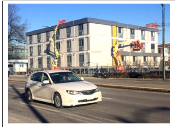
Figure 17: Modular housing units installed
