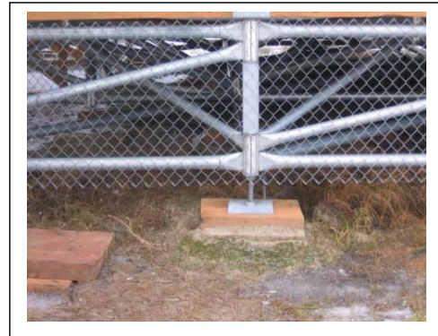
Figure 8: Typical base support on larger timber pads.
