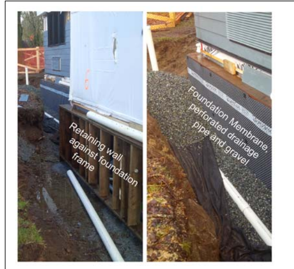
Figure 19: Retaining Wall at Foundation
